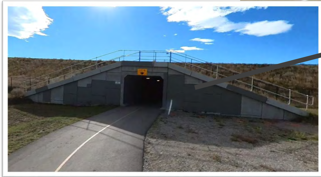
*Example pedestrian tunnel
